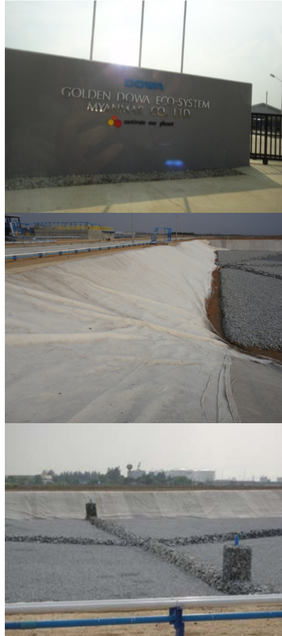
Figure 8: Dowa industrial waste treatment facility in Yangon. Source: authors, 2016
